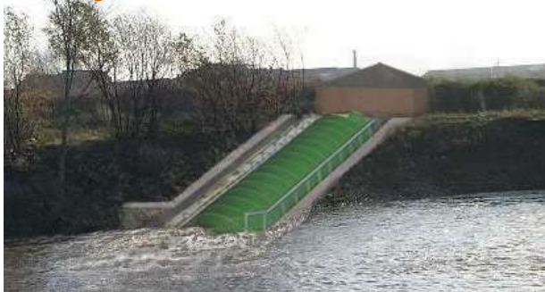
Project 1 – Jordan Dam
